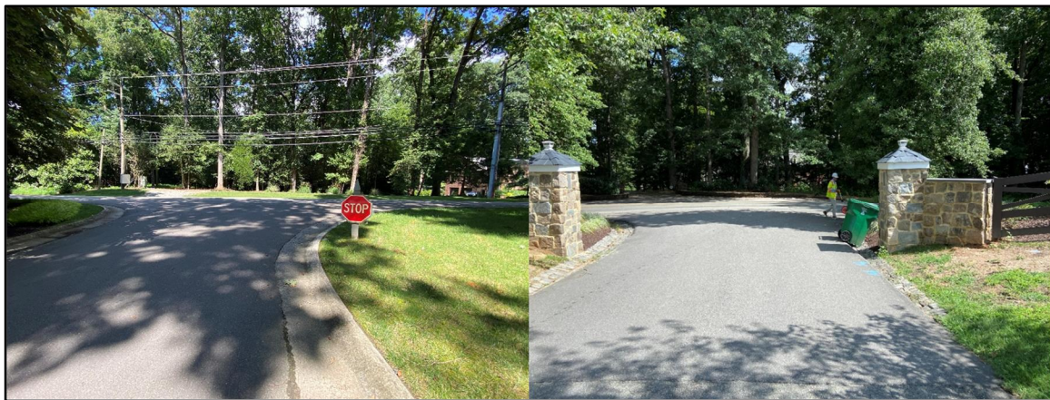
Photograph 1: Non-Compliant and Deficient Minor Street Signs
